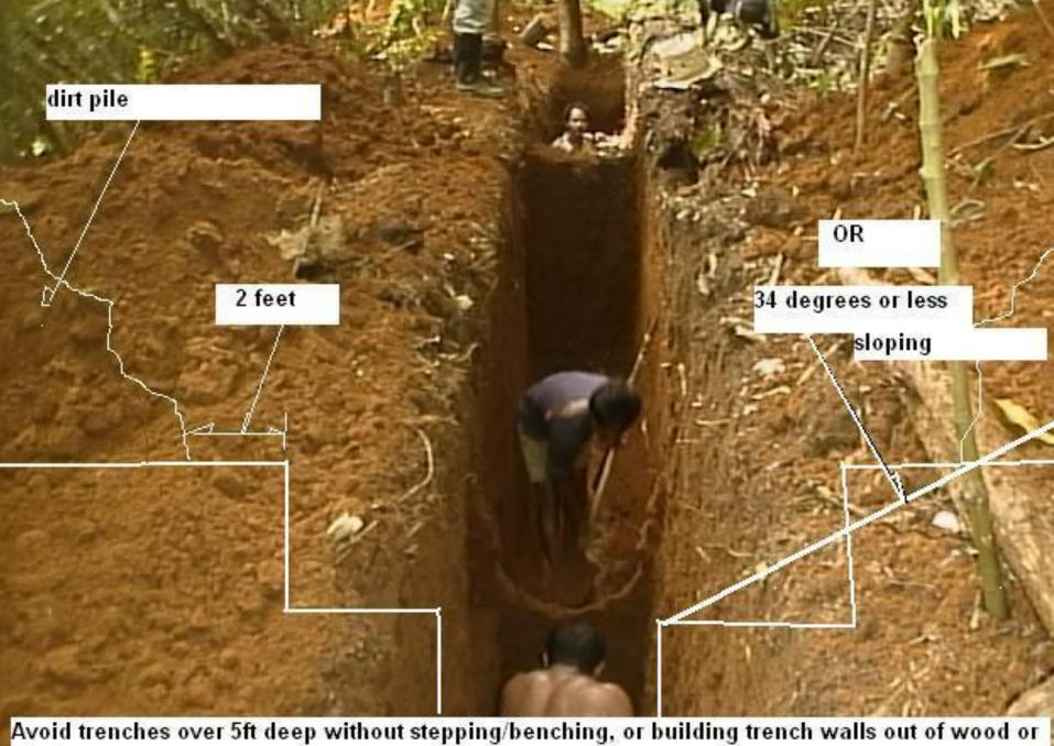
Avoid trenches over 5ft deep without stepping/benching, or building trench walls out of wood o steel
