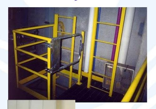
1910.28(b)(3)(iv) - Each employee is protected from falling into a ladderway floor hole or platform hole by a guardrail system and toe-boards erected on all sides, except at the entrance to the hole, where a self-closing gate or an offset must be used
